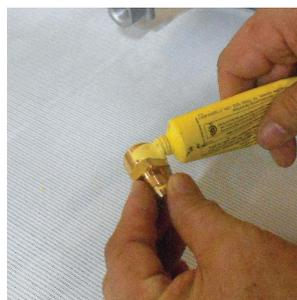
Apply gas pipe sealant all the way around the Flair Adapter's thread that will connect to the Natural Gas Valve
