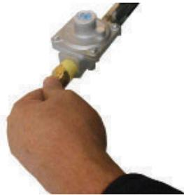
**Screw orifice into natural gas regulator**
