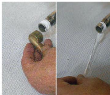
Remove propane valve and then teflon tape from the thread
